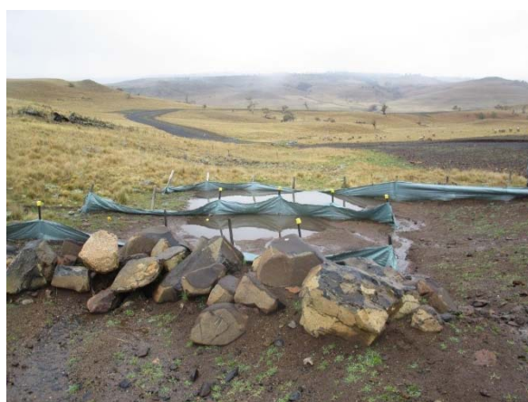
Photo 3 – installation of rip rap uphill of the larger rocks would assist in slowing water and would improve function of the sediment pond system
